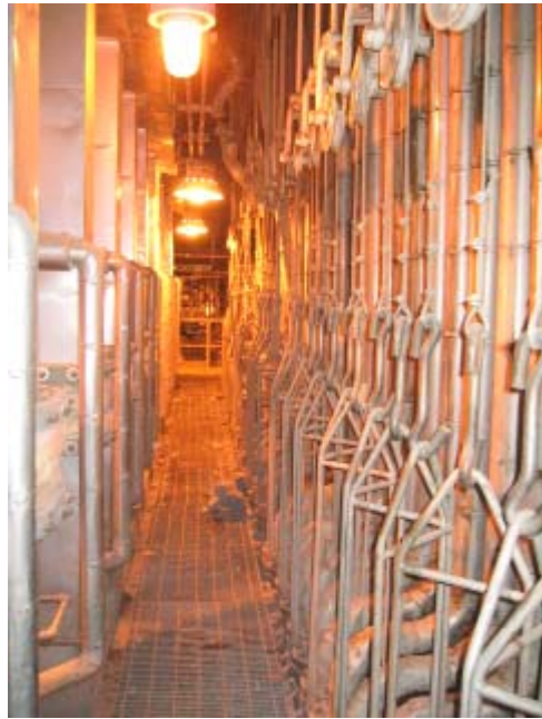
Photo 2 - Pre incident general radiant tube arrangement
