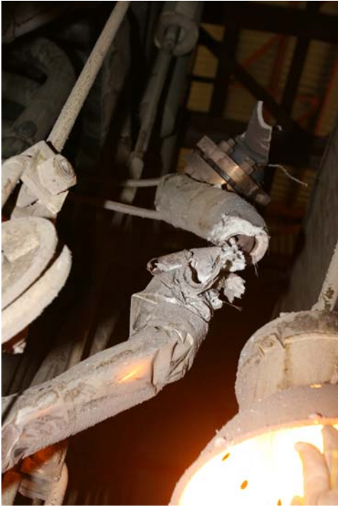
Photo 5 - Tube 161 lifted approximately 16 ft (view looking up)
