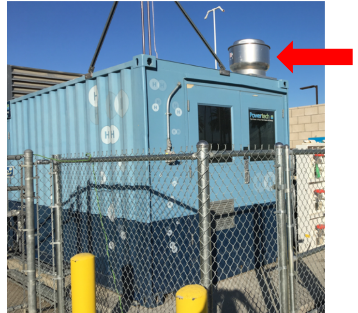
Compressor HEE with mechanical ventilation
