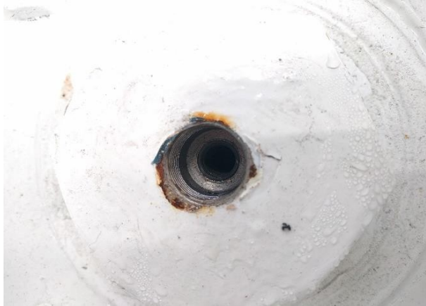
Figure 9: High-pressure tank port. Insert a 9f16" copper seat saver here
