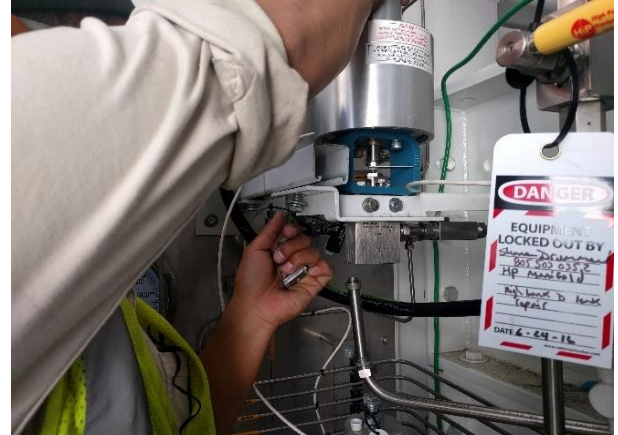
Figure 10: Reinstall of AOV105 assembly. Be careful to support assembly during reinsertion of cone and thread connections.
