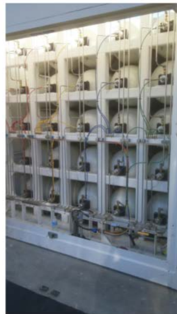
25x medium pressure hydrogen storage cylinders
