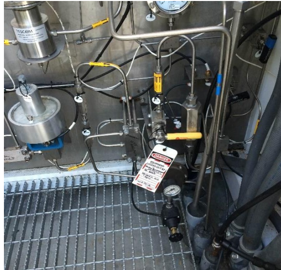
Figure 2: Compressor suction valved out, LOTO'd
