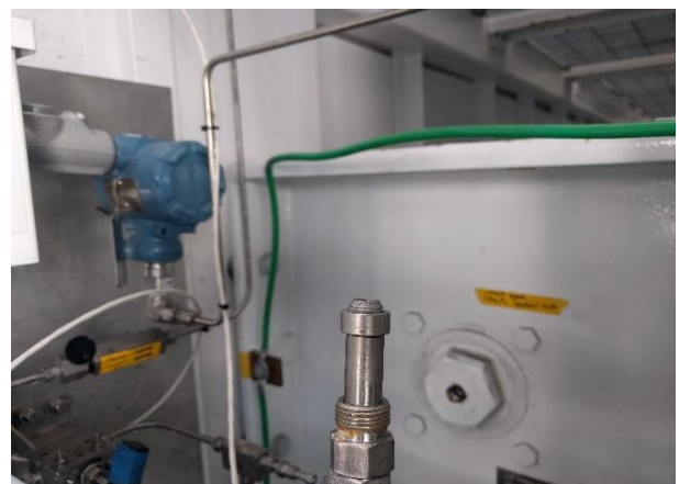
Figure 8: In this case the problem was most likely the fact that there was only about one thread assembly showing on this cone and thread fitting
