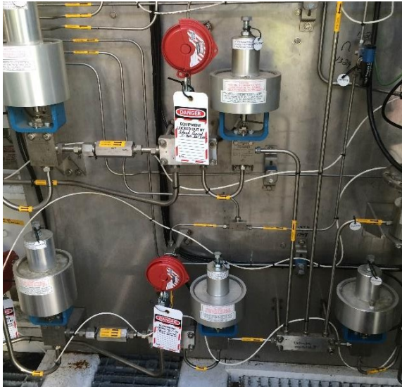
Figure 5: Location where high-pressure tube pressure transducers get their reading. They are shut in order to prevent false purge reading. They are also LOTO'd
