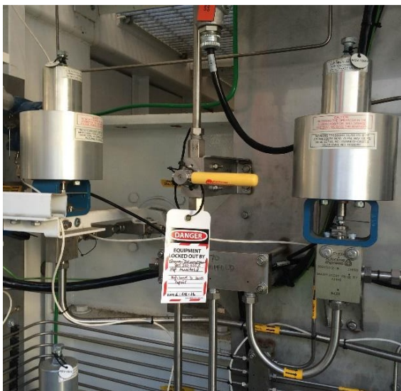
Figure 3: Compressor discharge valved out, LOTO'd
