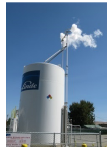
Figure 1: LH 2 Venting
