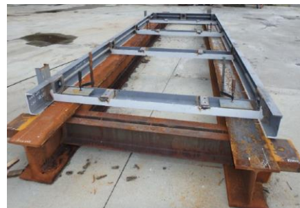
(b) Steel frame (top part)
