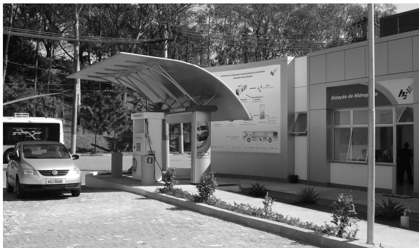
Figure 1. View of the front of the Hydrogen Fueling Station, operated by BR Distribuidora and located at EMTU/SP, São Bernardo do Campo.
