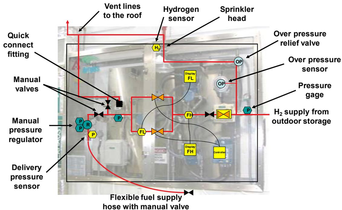
Figure 3: Hydrogen distribution panel [10]
