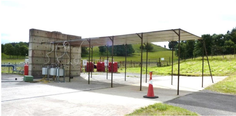
Figure 4: Ceiling Construction Over Release Point
