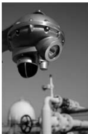
Figure 9. Ultrasonic leak detector above gas piping (from Gassonic) [16].
