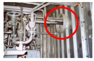
Figure 5. Gas Pipe in Ventilation Duct
