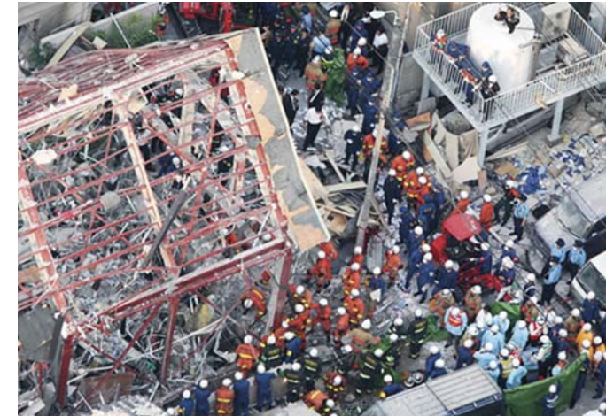
Gas explosion accident at the hot spring facility (2007, Japan)
