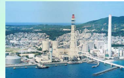
Energy plant (Coal-fired power generation plant)
