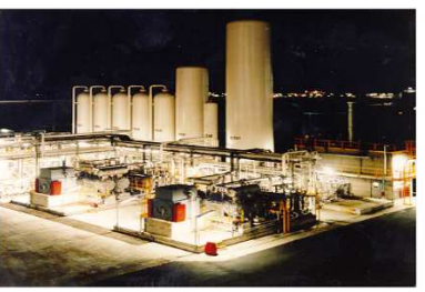
SMR, Electrolysis purification, liquefaction
