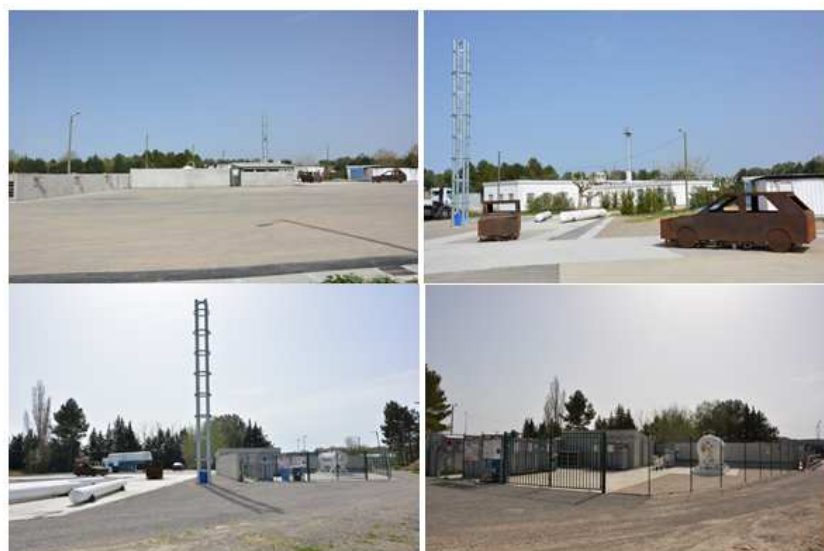
Figure 1. Photos of ENSOSP's operational training facilities.
