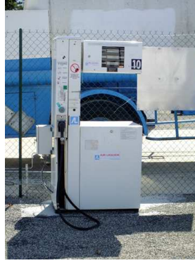
Figure 13. Mock-up hydrogen dispenser at the refuelling station training platform.
